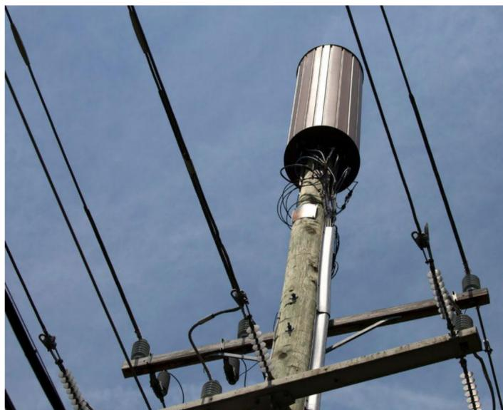
5G small cell mounted on power line
